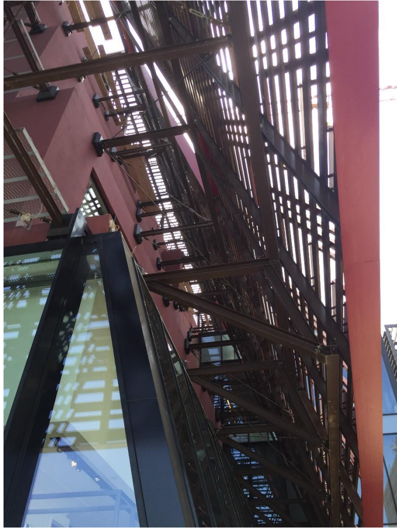
Bottom View of the building envelope
