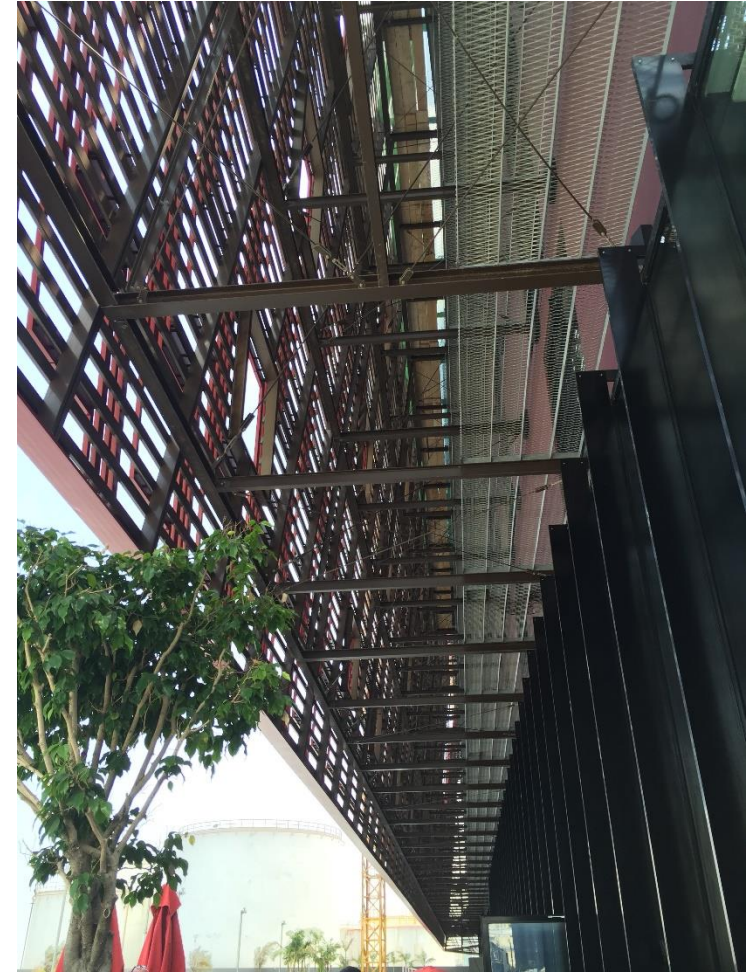
Bottom View of building envelope
