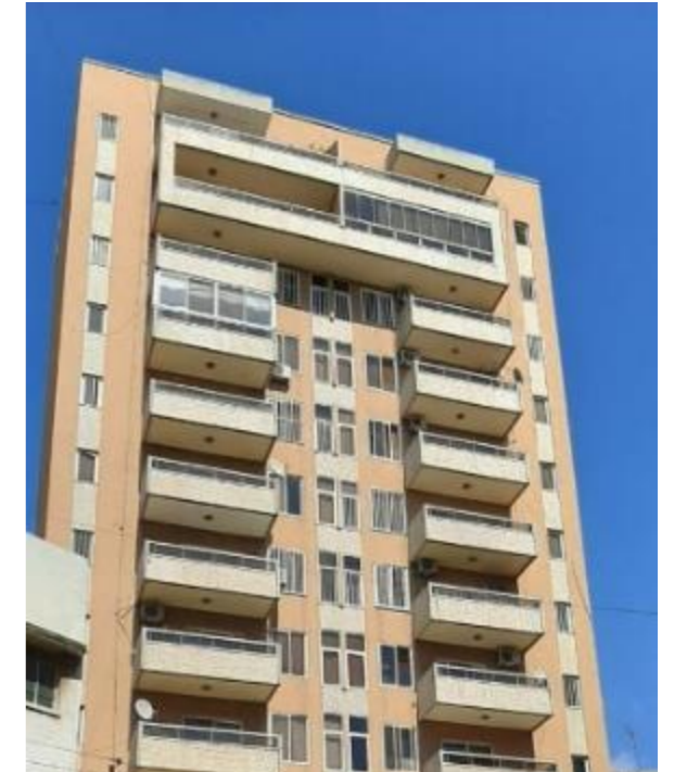
15-story multi-family home, as is typical of new constructions for larger developments.
