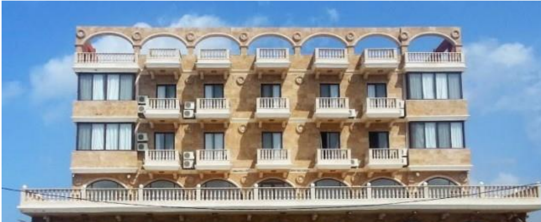
Six-story multi-family house with one attached wall as often constructed in the urban centres of the MENA region.
