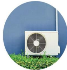
Condensate Capture 3-4 Liters of water directed to STP
